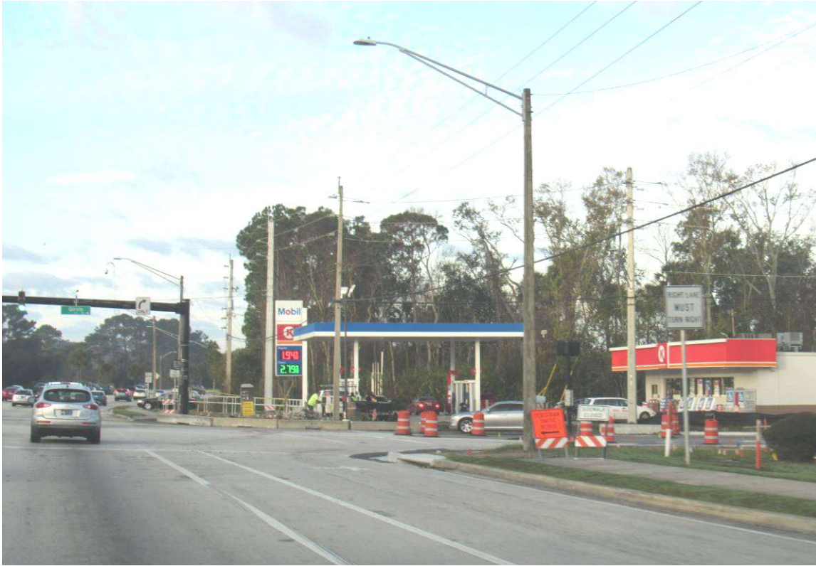
View of existing filling station
