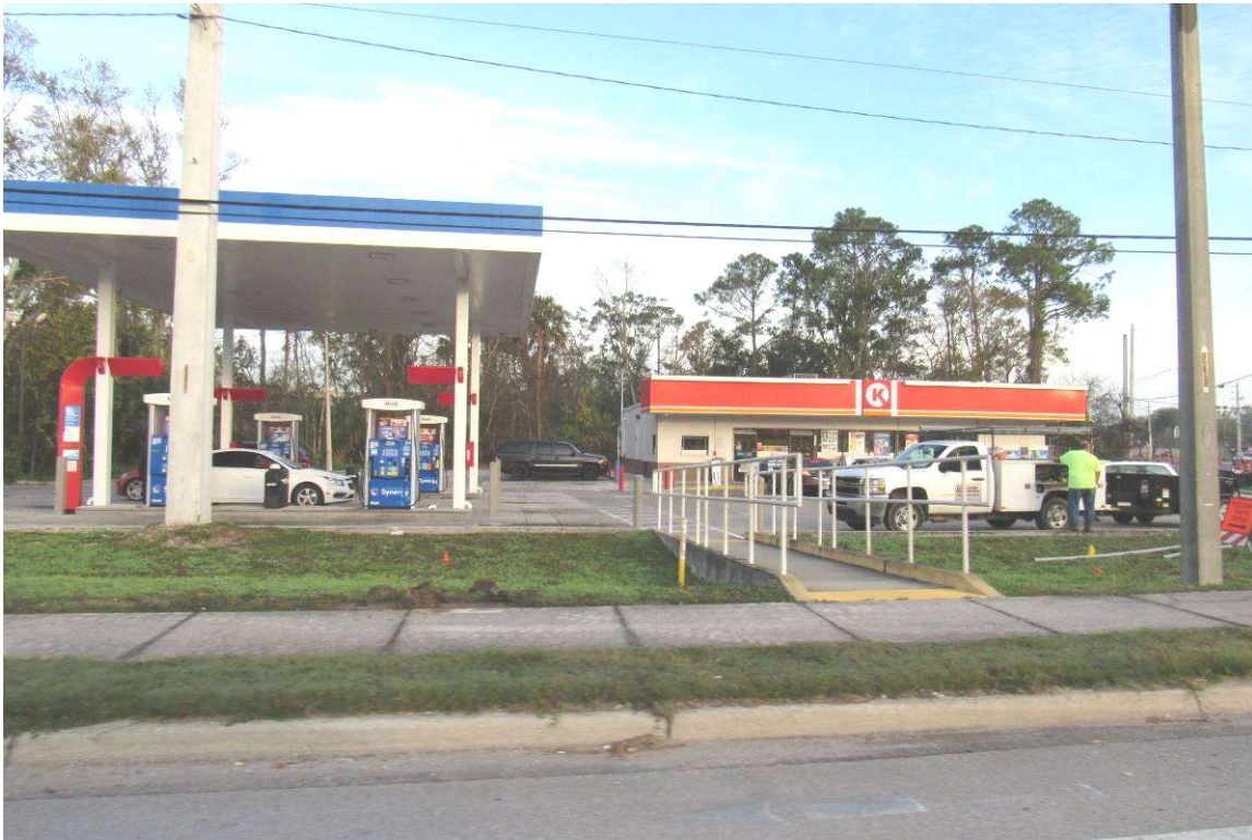
View of existing filling station
